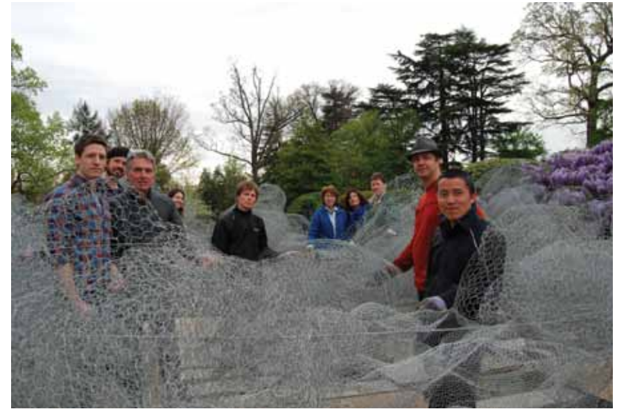
Andy Cao with the construction crew of Cloud Terrace on the Fountain Terrace, spring 2012.
