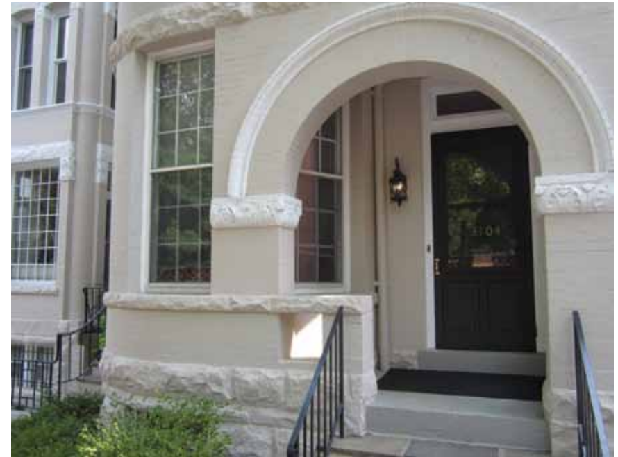
The Oaks townhouse reopened for visitor and staff use when renovations were completed in August 2011.
